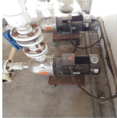
Energy efficient multistage monoblock pump
